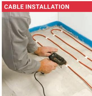
Clean the floor. Apply a layer of adhesive primer. Attach the cable (eg. use glue gun) on the floor.
