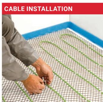
Determine the position of the heating zones before starting the installation of the heating cable and screed layer in agreement with the planner/architect. Attach the cable on a metal mesh (with KBL-10 cable ties) using the desired cable spacing.
