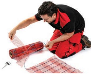
net band also allows for quicker installation of underfloor heating in irregularly shaped rooms.
