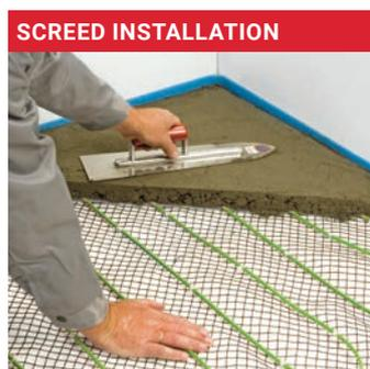
Carefully apply a screed on top of the cable. Let it cure according to the manufacturer's instructions. Depending on the type of screed this process can start after 7 days (anhydrite screed) or 21 days (cement screed). The first heating up and down procedure of the screed has to be agreed with the supplier and documented.
