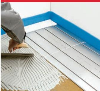
Apply Reflecta Adhesive A-FIX onto the subfloor (or use 15 screws per plate for wooden subfloors). Place the Reflecta plates on top of the glue.
