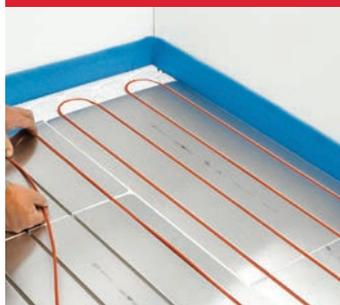
Place the T2Red heating cable into the grooves. The desired heat output is determined by the spacing of the cable.
