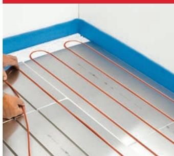
Place the T2Red heating cable in the grooves. The desired heat output is determined by how closely you space the cable (100, 200 or 300 mm).
