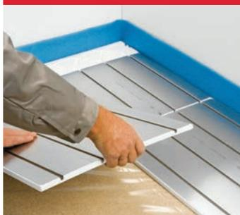
Lay out the Reflecta plates (no need to screw or glue them) on the subfloor.
