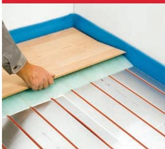
Place a wood floor underlay on top of the Reflecta plates and then lay the new wooden or laminate floor according to the instructions of the manufacturer.
