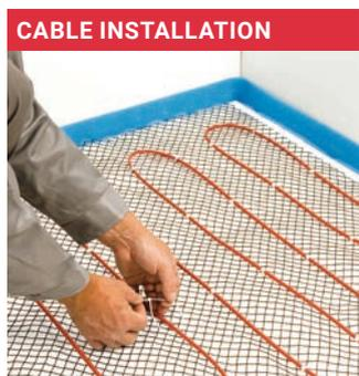
Determine the position of the heating zones before starting the installation of the heating cable and screed layer, in agreement with the planner/architect.
