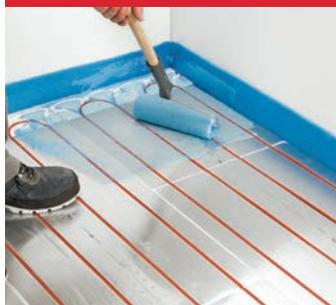
Apply the Primer P-Fix on the aluminum layer.
