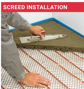
Carefully apply a screed on top of the cable. Let it cure according to the manufacturers' instructions. Depending on the type of screed this process can start after 7 days (anhydrite screed) or 21 days (cement screed). The first heating up and down procedure of the screed has to be agreed with the supplier and documented.
