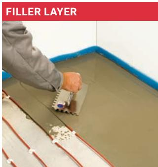
Carefully apply an even layer of filler on top of the cable. Let it cure according to the manufacturers' instructions.
