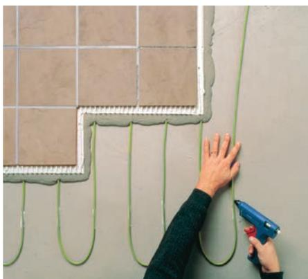
The flexible underfloor heating cable is suitable for very well insulated properties installed directly in a levelling compound.
