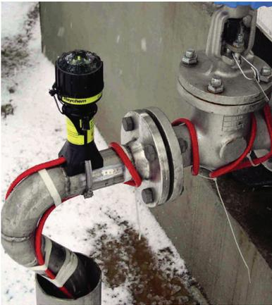
When comparing the total installed cost, total operating cost and total maintenance cost - electric heat-tracing systems are typically your best overall value.
