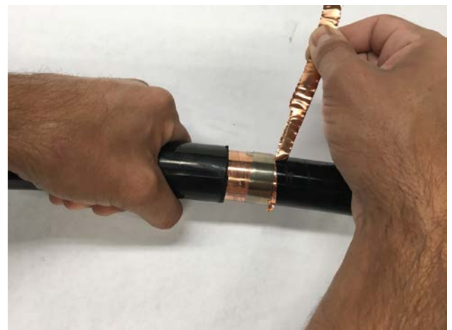
Figure 3: Using the roll clip to cut and remove the copper screen
