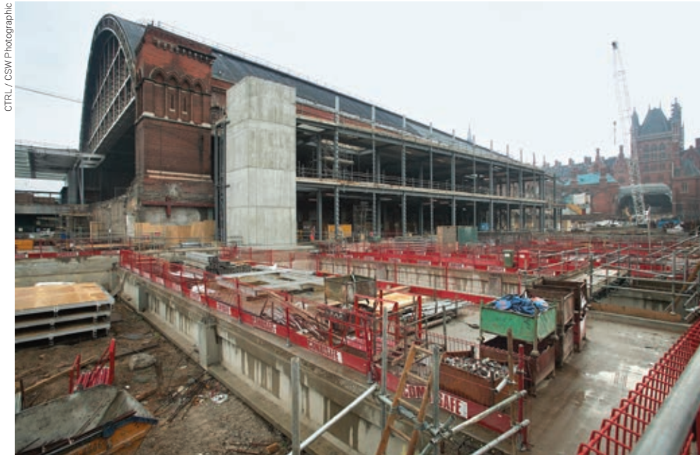
Work on the Thameslink Box outside of St. Pancras Station.
