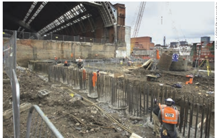
Piling work being completed outside of St. Pancras Station.
