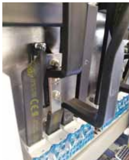
MTO nVent ERIFLEX Flexibar Advanced shaped: Twist, Bend, Fold
