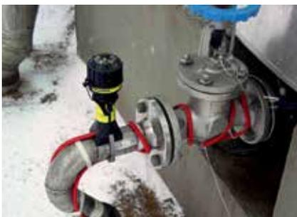
heating cables, etc. As each cable type has its own features, functions and benefits, we provide expertise to identify the most appropriate solution optimised to the specific needs of the plant or application.
