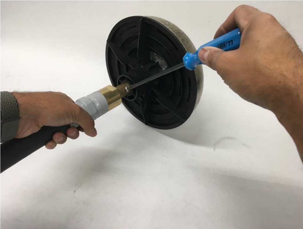
Figure 15: Once the nVent ERICO DYNASPHERE has been fitted to the termination coupling, ensure the locking screw is tightened securely
