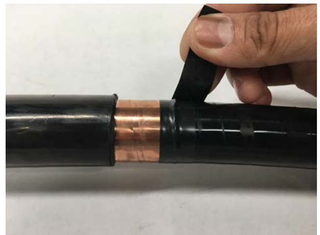
Figure 4: Placing PVC tape to prevent further unraveling
