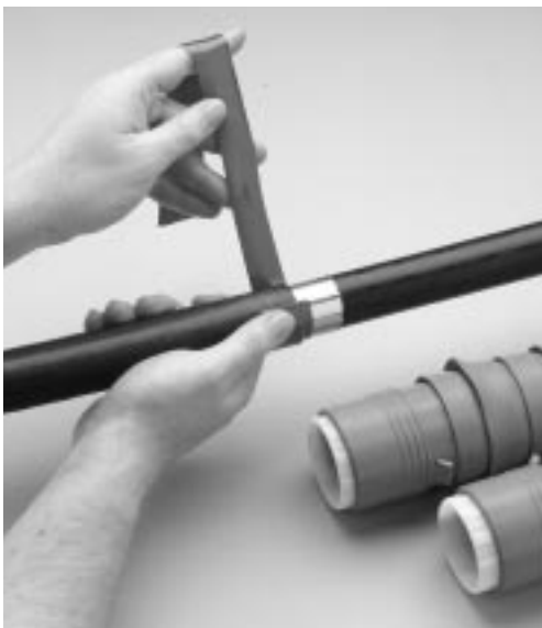
Photo 4: Red sealant tape applied over overlap.
