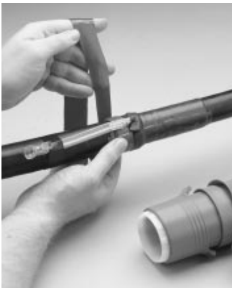
Photo 7: Apply the sealant tape below the stress control patch.
