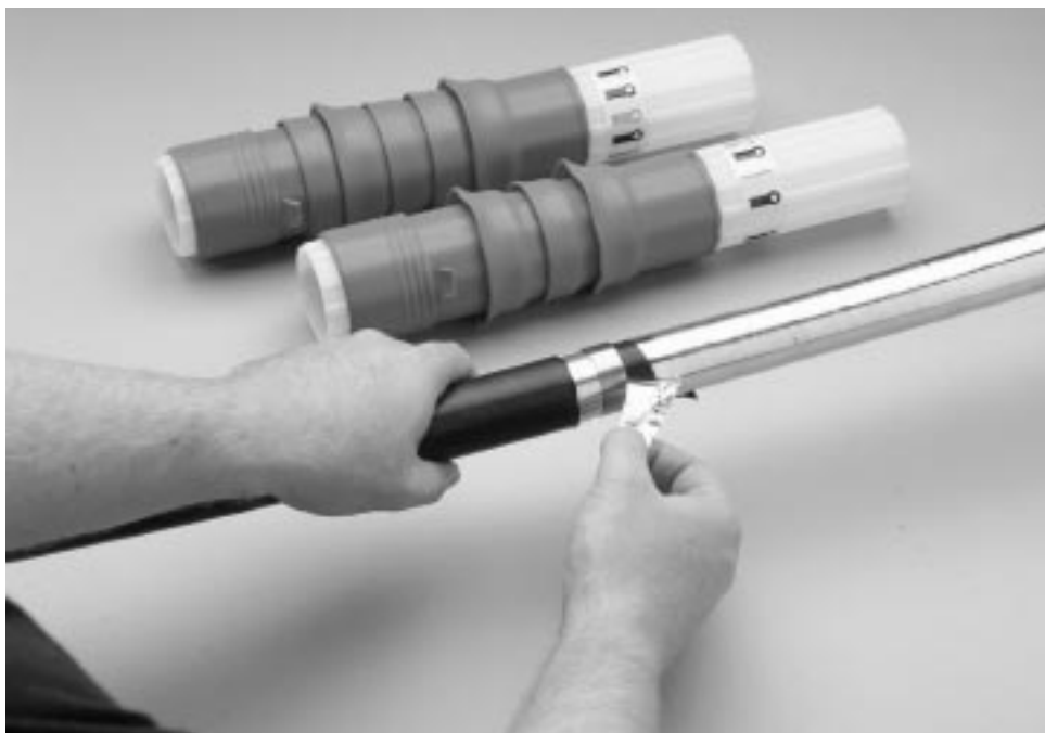
Photo 3: Using the roll clip to cut and remove the copper screen.
