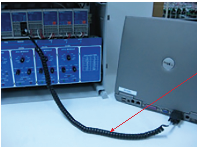
RJ-11 to 9 pin D-Sub female cable used to connect the NGC-40 to your computer
