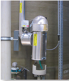
Heat-tracing installation
