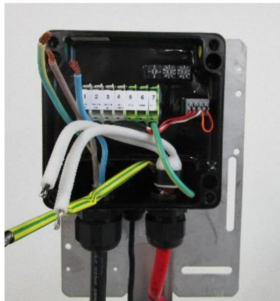
12/ Connect the power cable to the cage clamp terminals. When needed remove the insulation of the power cable conductors a bit further to ensure good electrical contact with the cage clamp terminals.
