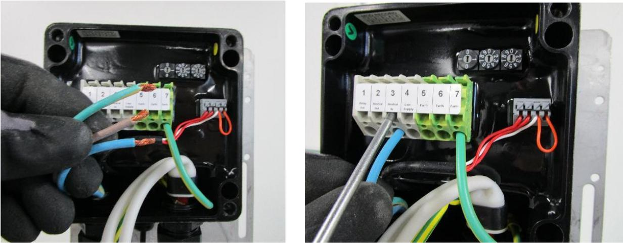
13/ Connect the heating cable to the terminals. To make sure the heating cable conductor is installed correctly in the cage clamp terminals slide the white insulation (= nVent RAYCHEM core sealer) back during the installation.
