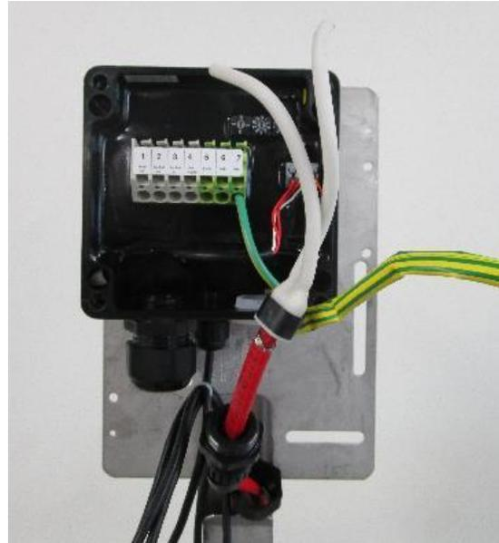
9/ Remove the temporary rain plug (white color) on bottom side of the enclosure.
