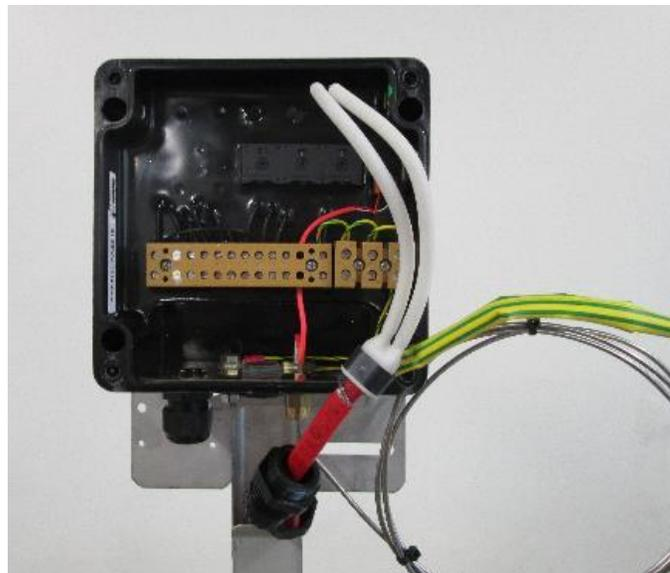
8/ Mount the ETS-05 thermostat on the same support bracket, after removing the front lid. The preferred mounting position is indicated on the picture below.
