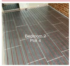
The nVent RAYCHEM T2Red cabling with self-regulating technology was chosen as the best system for the project, providing peace of mind that no hot spots would occur and providing great flexibility as it can be cut to length on site.
