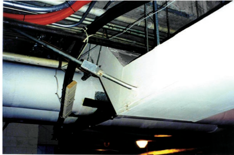
Figure 10. Inadequate Cable Penetration of Fire Protection Enclosure
