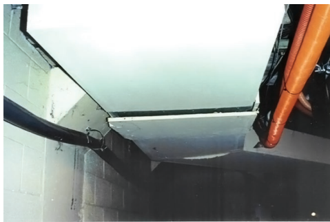
Figure 11. Improper Gypsum Board Enclosure Installation
