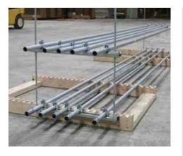
The spacing between conduits across the channel needs to be the same so that they meet up with each other when the individual runs are installed. It is recommended that installers use custom wooden jigs with notches at the spacing for each piece. They can be easily made on the jobsite with pieces of wood and customized for individual situations.
