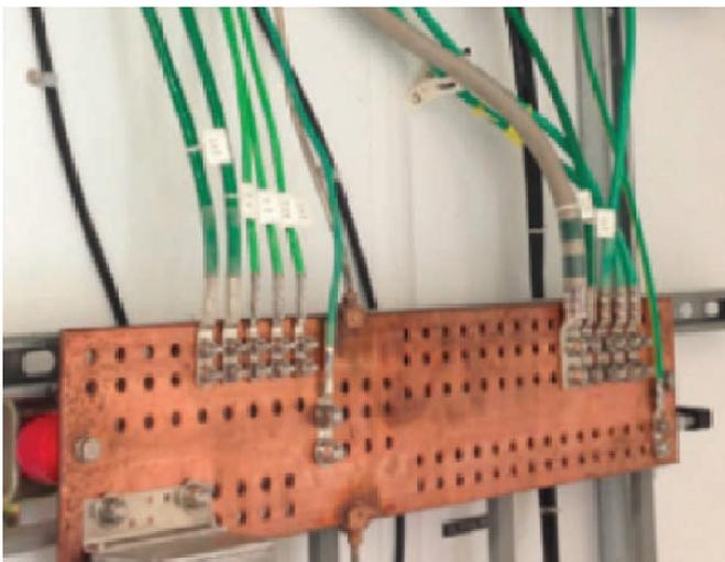
Figure 3: Typical Single Point Connection Window
