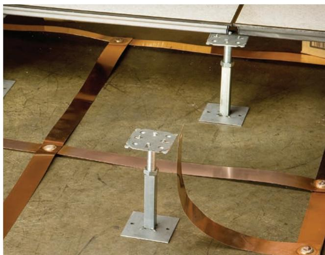
Figure 4: Examples of Bonding Mat or Signal Reference Grids
