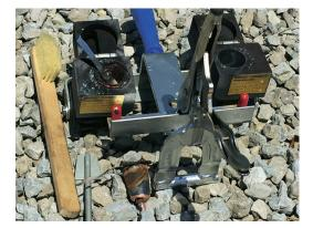
Open the mold and remove the expended steel cup - no special disposal required.
