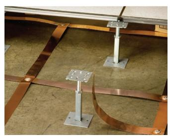
Figure 4: Examples of Bonding Mat or Signal Reference Grids
