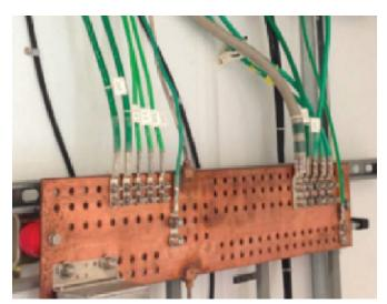
Figure 3: Typical Single Point Connection Window
