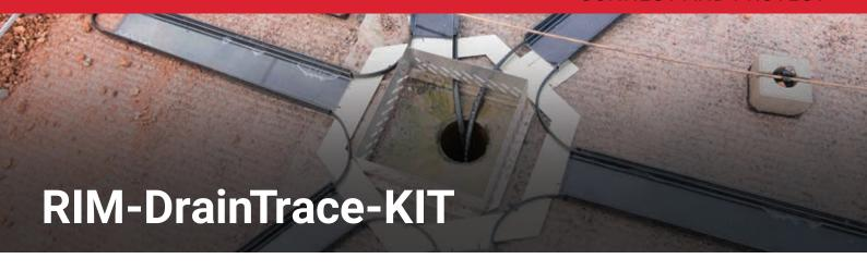
The **nVent RAYCHEM RIM-DrainTrace-KIT** provides an **all-in-one solution** to keep your roof drain snow and ice free, avoiding any unpleasant surprises due to snow and ice build up during the toughest winter period.
