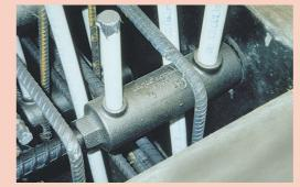
Standard 1/2" (13 mm) and 3/4" (19 mm) PVC or flexible tubing is used for the inlet and outlet ports.
