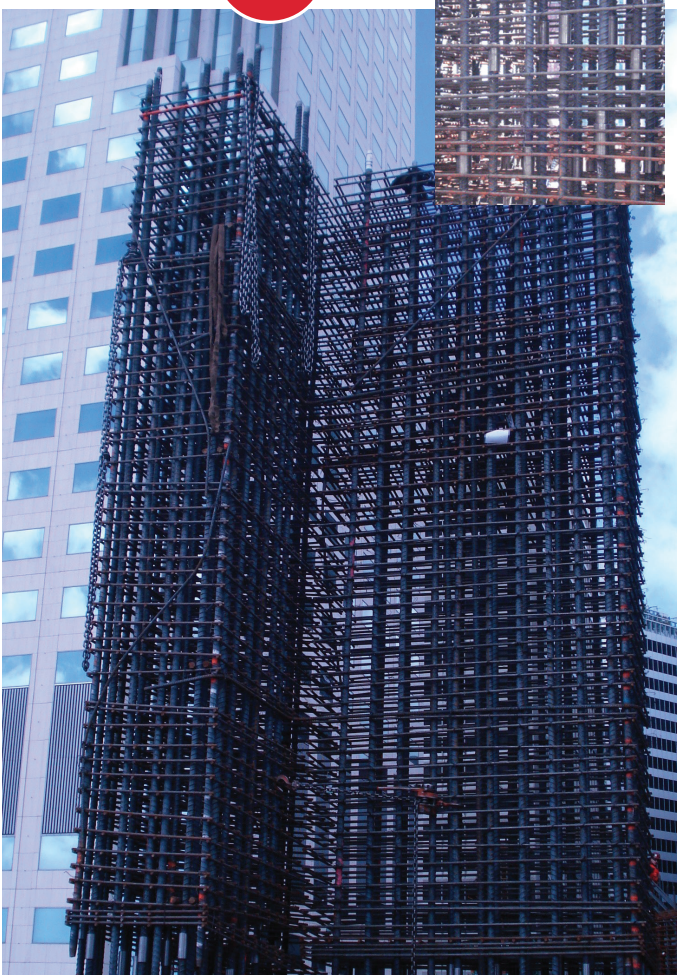
Mechanical splicing reduces congestion
