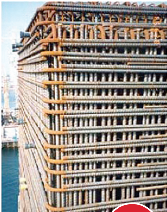
Lap splicing produces congestion
