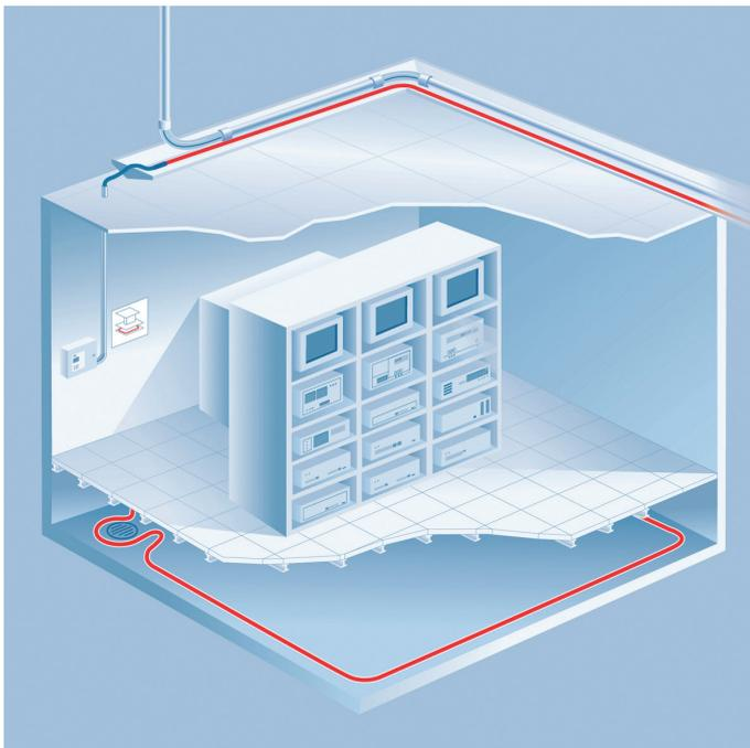
Furnish a complete system, including digital electronic alarm and locating modules, modular sensing cable/water detection probes, map, and auxiliary equipment as manufactured by nVent and known as the nVent RAYCHEM TraceTek leak detection and location system.
