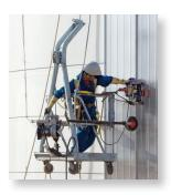
To meet the needs of this application, nVent employed its Trac-Loc insulation system which is an advanced interlocking panel system consisting of prefabricated panels of insulation and jacketing material, in this case mineral wool & stucco-embossed aluminum.
