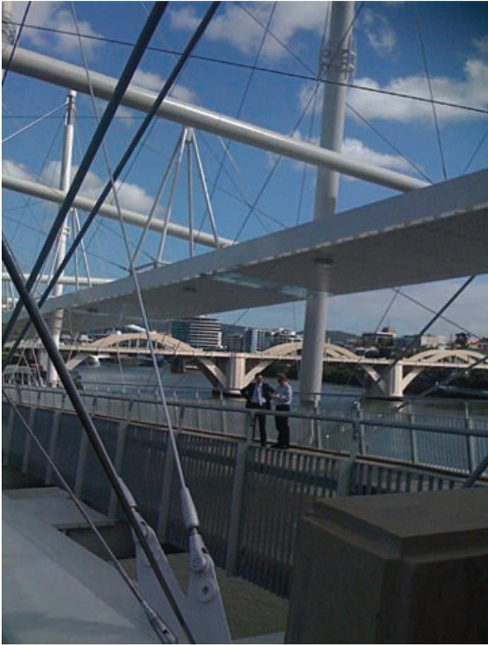
The Kurilpa Bridge is the world's first tensegrity pedestrian and cycle bridge.
